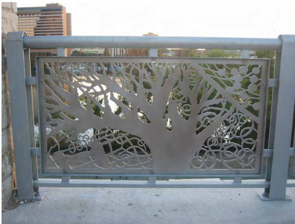
Public art was incorporated into the recent Cesar Chavez sidewalk reconstruction.
