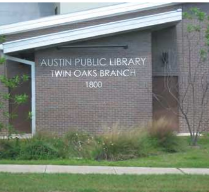
The Twin Oaks Library in the Bouldin neighborhood, which opened in 2010, incorporates green building principles.
